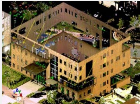
The yellow arrows indicate where the building's black-colored windows should be. These darkly colored and translucent features were not captured with laser scanning.
