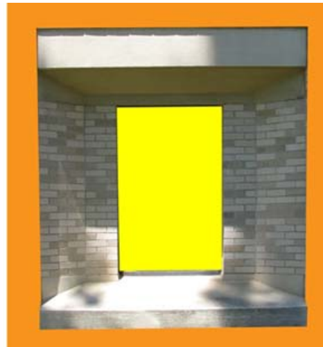
Figure 8 (Left) Complex window to be modeled (Right) Familiarize yourself with the layers of space to be modeled – here yellow represents the farthest plane (the glass) and orange represents the closest plane (the wall in which the window is set)
