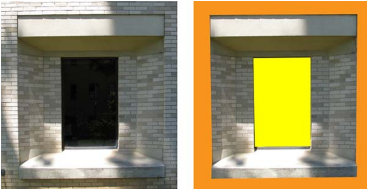
Figure 8 (Left) Complex window to be modeled (Right) Familiarize yourself with the layers of space to be modeled – here yellow represents the farthest plane (the glass) and orange represents the closest plane (the wall in which the window is set)
